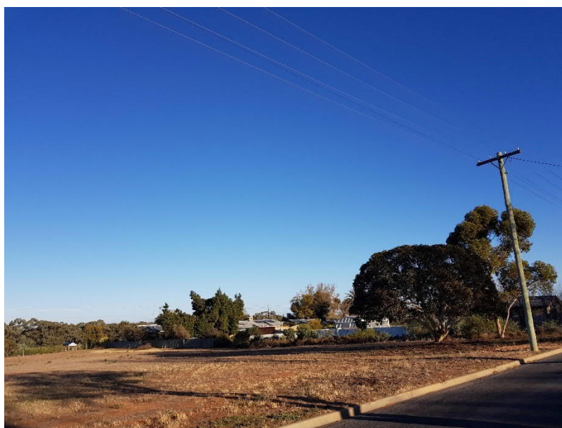
Photo 4 – Existing powerlines on Friel Street
