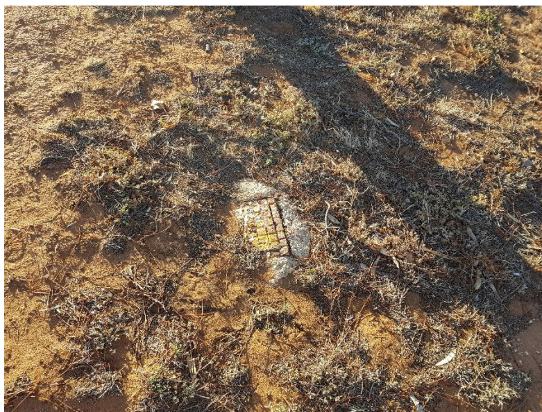
Photo 3 – Typical fire plug
