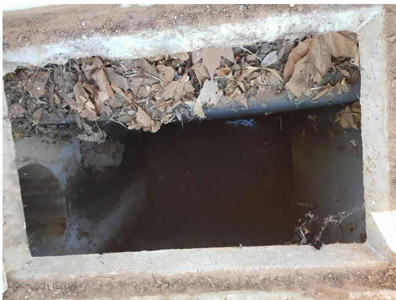
Photo 2 – Stormwater pit at southeast corner of site
